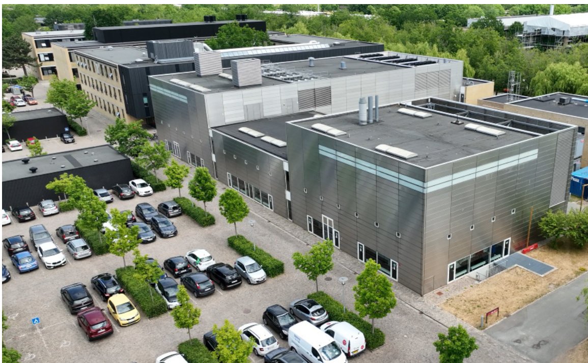
B346A IS BEING BUILT AT ØRSTEDS PLADS. Nanolab Phase 4 will be built on Ørstedes Plads on the DTU Lyngby Campus and will be connected with the existing clean room, so that a unified facility is created. Photo: DTU
