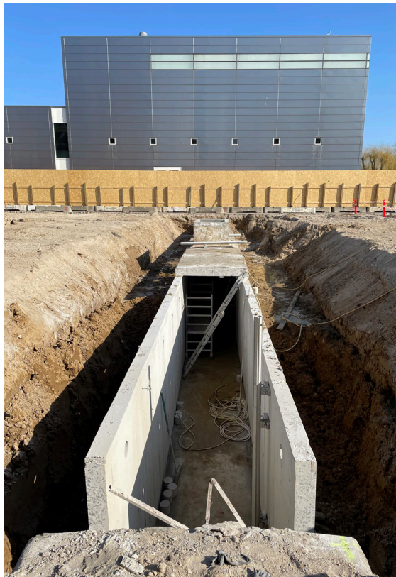
The tunnel system beneath DTU is over 50 years old and serves as a vital supply line for Lyngby Campus. Part of the site preparation at Ørstedes Plads involves removing a section of the old tunnel and constructing a new one. Photo: DTU
